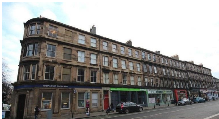
Figure 1- 51-77 South Clerk Street (Historic Scotland, 2022)
